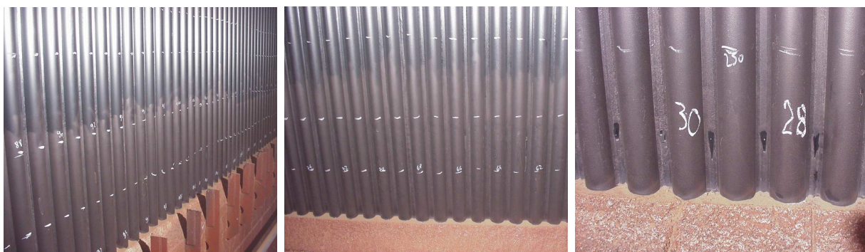
Figure. 5. Water walls after one year exploitation, OFz-425 I - Siersza Power Plant
