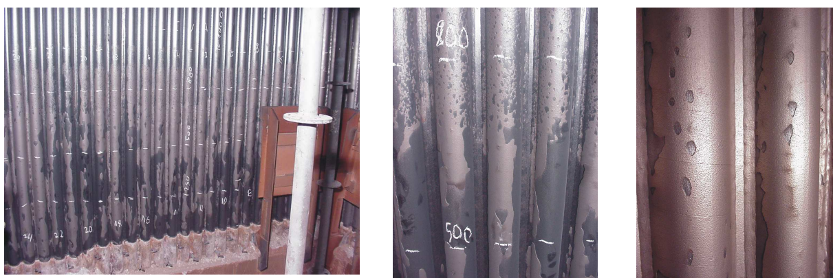
Figure 2. Water walls after one year exploitation, OFz-450B Żerań. Coatings sprayed by M-S
