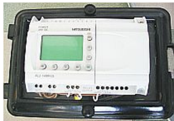
Fig. 8. Control unit of the lift with Alpha XL mounted on top of the box.
