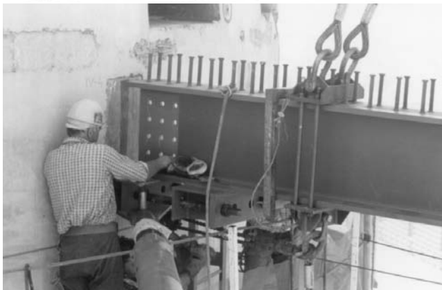
Fig 1. A view of a joint of a steel beam and a composite reinforced concrete structure; 1 – a composite reinforced concrete core of the tower, 2 – an insert plate, 3 – backing distance of plate girders, 4 - plate girders of screw joints, 5 – a steel beam
