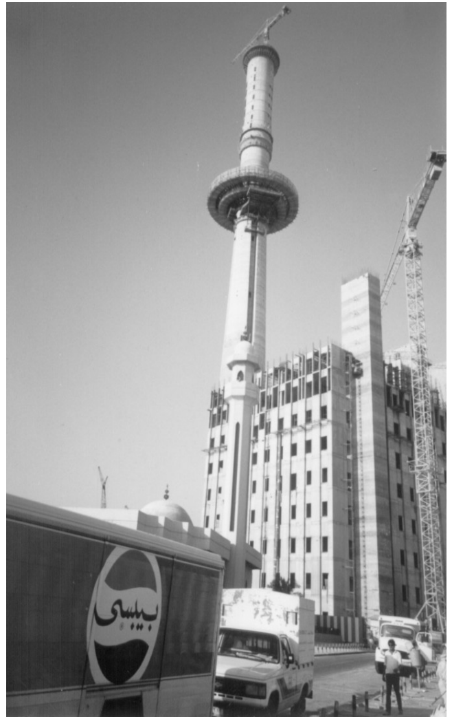
Fig. 2. The telecommunication tower in Kuwait at the stage of assembling of the steel structure
