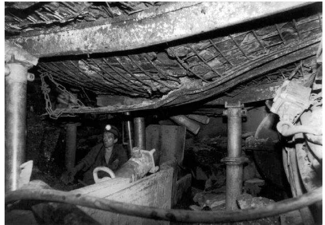
Fig. 7. Work in a wall pit
