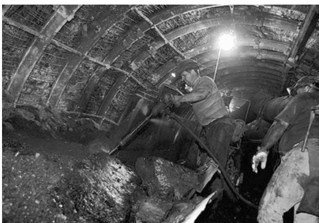
Fig. 6. Work in a corridor pit
