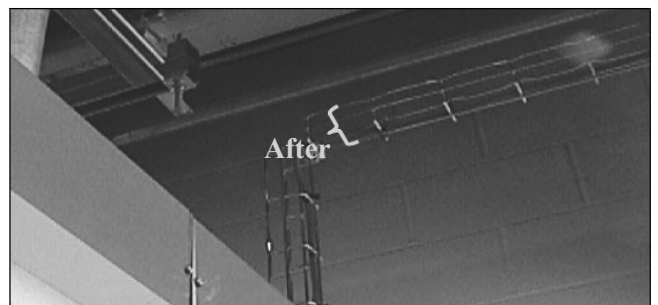
Fig. 4. Field wiring after Profibus technology (Courtesy Emerson Process Management)
