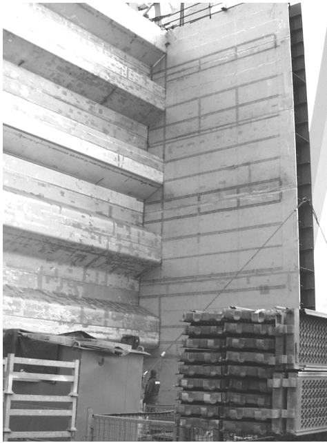
Fig. 8. A section of the tank welded using the FCAW method during assembling on a slipway [22]
