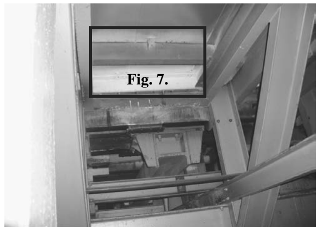
Fig. 6. The actual picture of testing area from a viewpoint of the following heating zones
