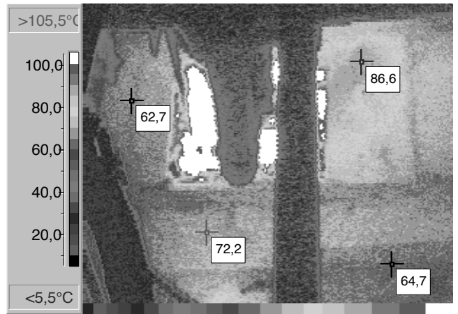
Fig. 5. The furnace roof, surroundings of burner diffuser no 2
