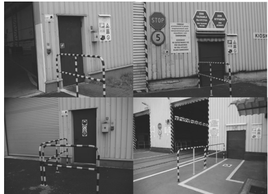
Fig. 8. Photography of security barriers in front of the entrances to the production buildings of the organization
