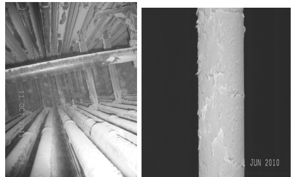
Fig. 2. Deposits on superheaters of the second pass on one of outlet pipes of the convection cage
