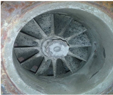
Fig. 6. Deposit on the turbocharger of a biogas engine formed by siloxanes
