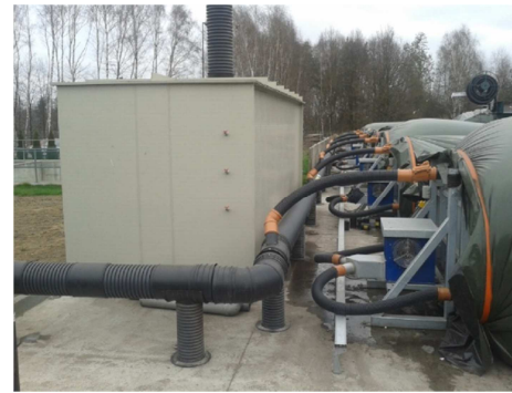
Fig. 7. Halloysite-based postprocessed air filter working in industrial-scale compost plant
