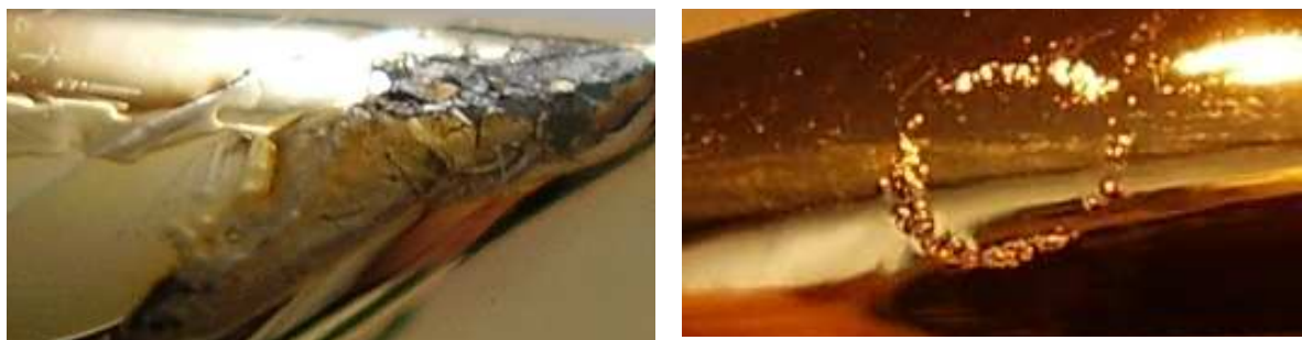
Figure 9. Corrosion points in a layer
